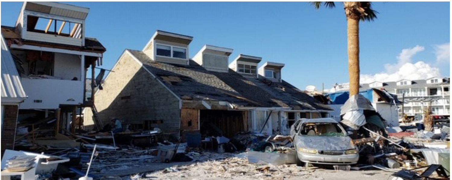
Figure 4. Devastation from Hurricane Michael resulted in damage to 80 percent of infrastructure for the City of Mexico Beach. AtkinsRéalis was on-site supporting within 10 days of landfall.
